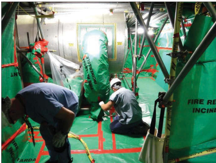
Left: Workers build an asbestos-abatement enclosure to protect the plant from contamination.
