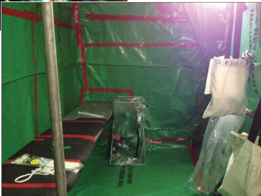
Below: The enclosure included a “clean” area, shown here, a shower area, and a “dirty” area, where the asbestos removal took place.
