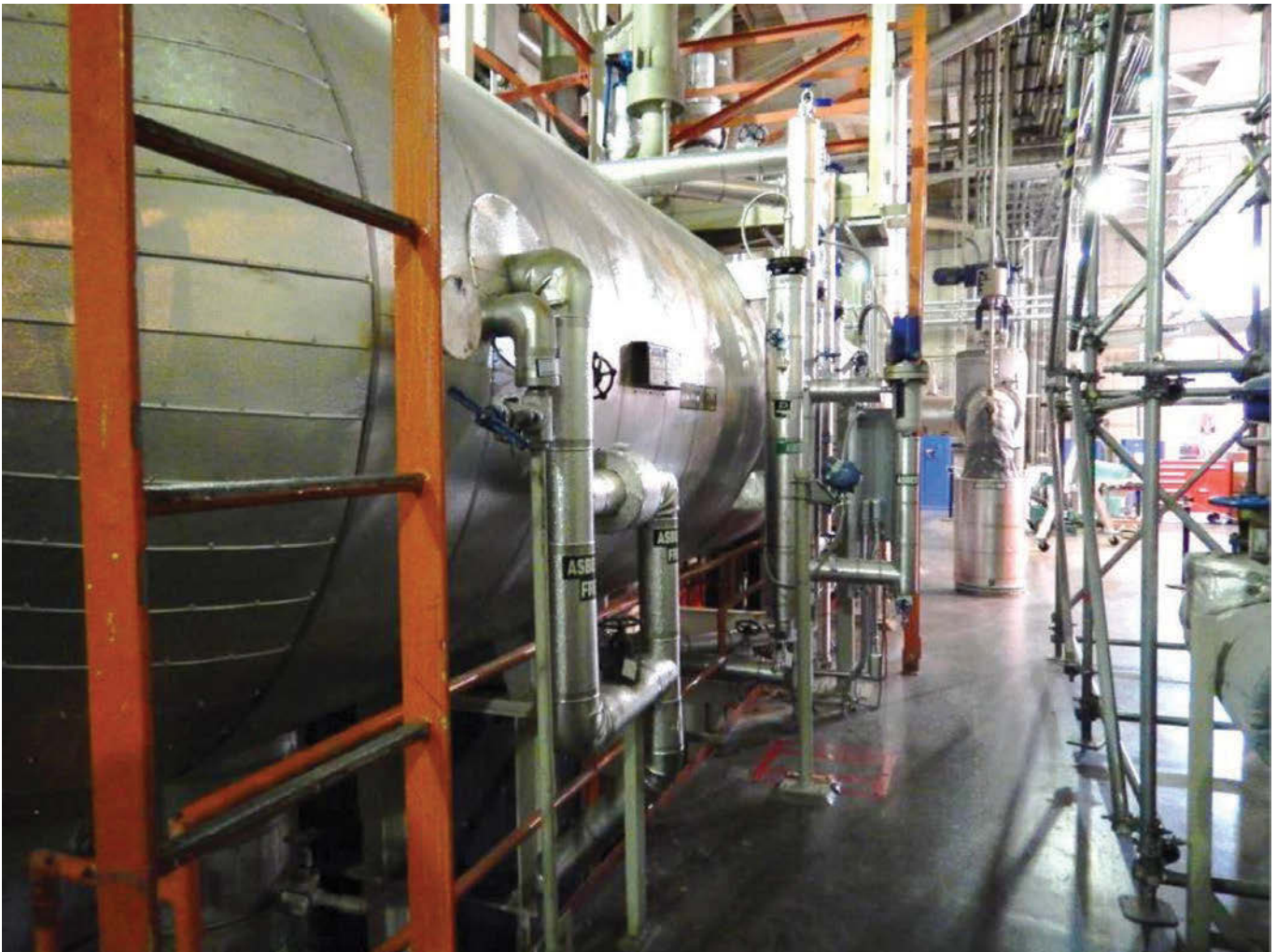
Unit 2's 6B feedwater heater after reinsulation
